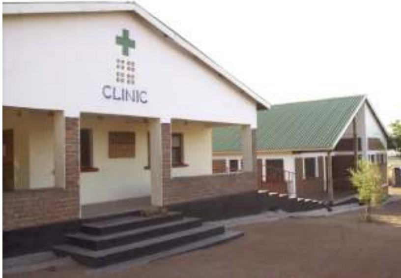
Original clinic building and new treatment unit
