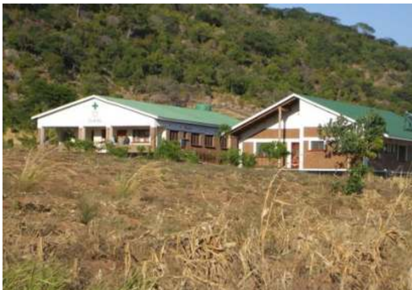
Original clinic building and new treatment unit
