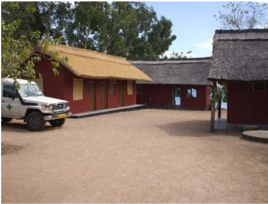
The new extension to the volunteer centre
